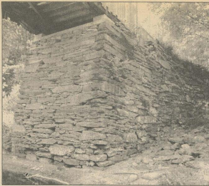
**This fieldstone abutment at the Downers Bridge in Weathersfield is one of the finest dry stone bridge foundations in the state.**
